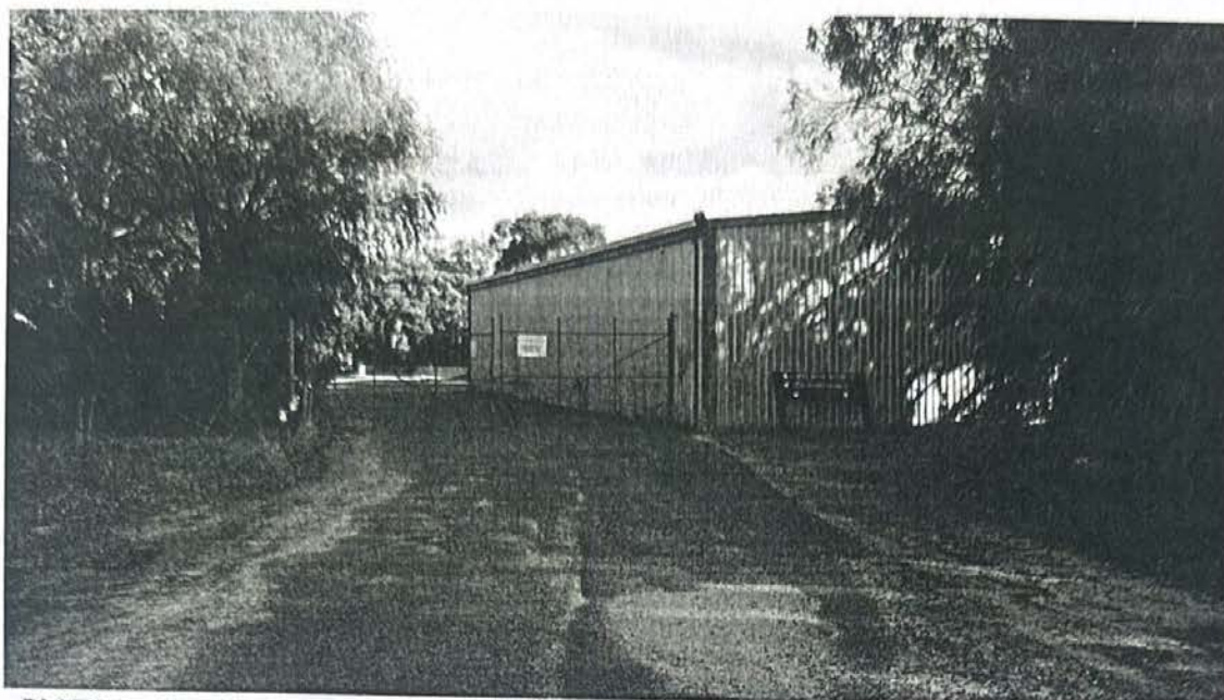
PLATE 1: City of Busselton Dunsborough Works Depot
