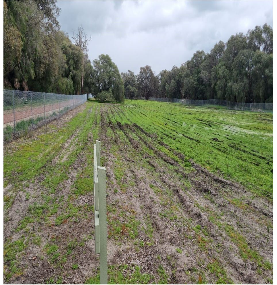
PLATE 24: Existing DBCA southern boundary fencing (September 2024)
